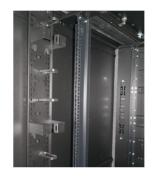
Horizontal Cable Management: metal and plastic cable organizer in different rack units, plastic finger cable troughs
